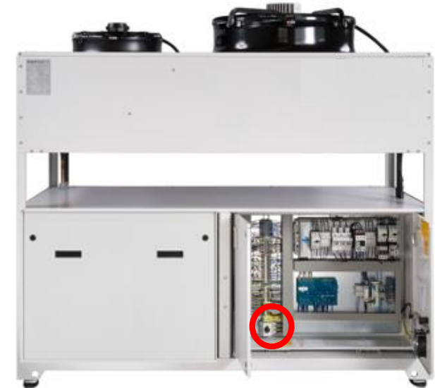
Turn off chiller power at "4Q1". It should be on the "0" position.
