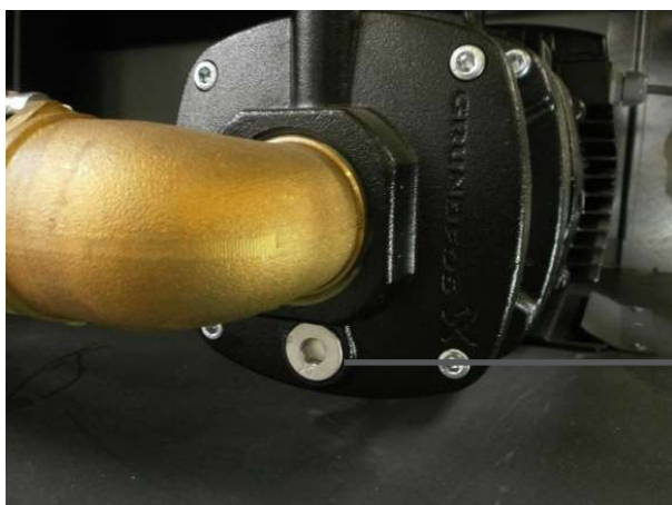
Figure 23: Position of the pump drainage (horizontal type)
