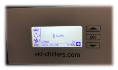
When the chiller is not in the faulted condition, the system will maintain cooling and display the activated components on the left side of the screen.
